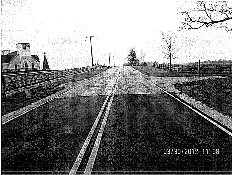
Transition from Big Rock Township Resurfacing Project
